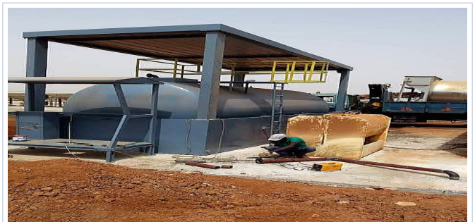
INSTALLATION Installation Gaz
